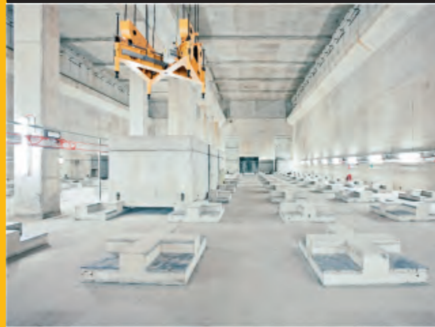
Inside the ILW store at Trawsfynydd
